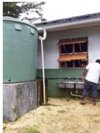
Photo Wash stations completed
