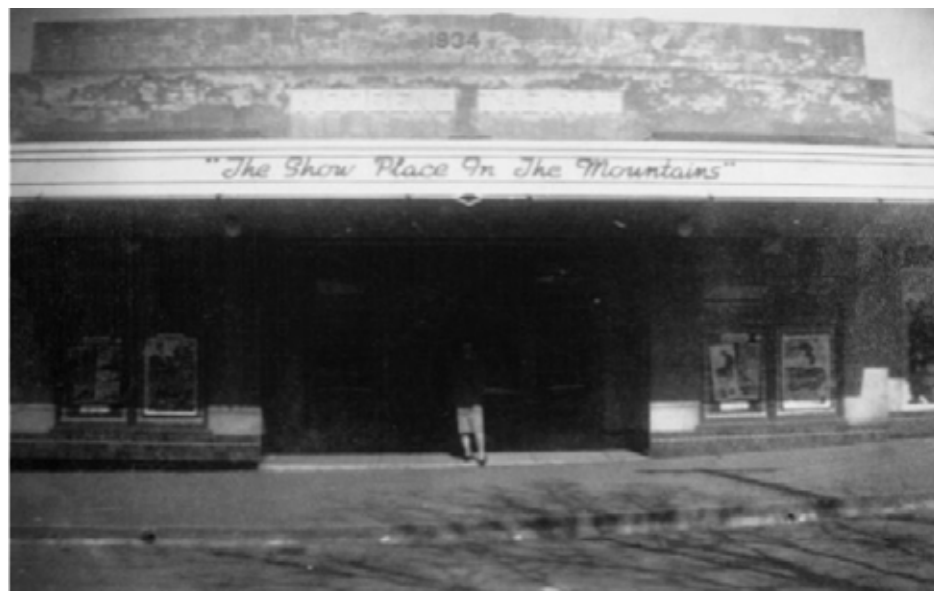
Photo 895: Woodend Picture Theatre. "The Show Place in the Mountains", High Street, Woodend. Note 1934 on top of the building. This is currently the only photo we have of the outside of the Theatre.
